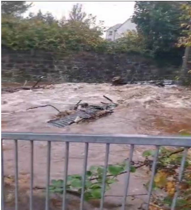
7 October 2023 – Left shows screen shot of video footage and the top of the automated screen with the complete submergence of the control cabinet behind.
